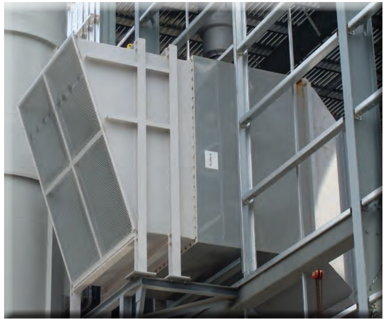
Major Design/Build firm for a Co-Generation Facility, Ontario Canada
